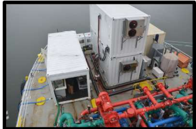
Installed on MERC Barge in Baltimore
